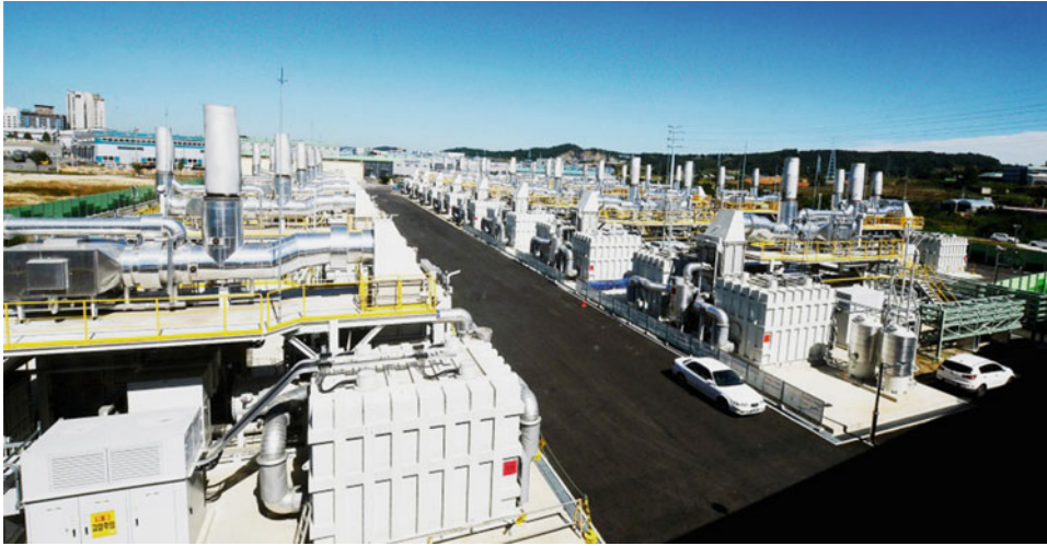
Abb. 6.44 59 MW MCFC – Gyeonggi Fuel cell park. (Quelle: Fuel Cell Energy [121])
